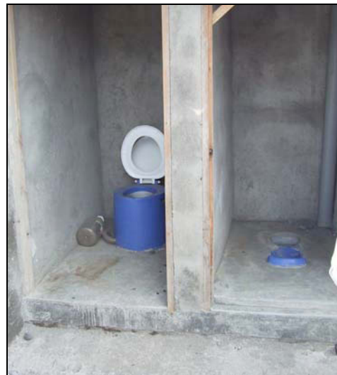
Figure 20 Construction of UDDTs in progress
