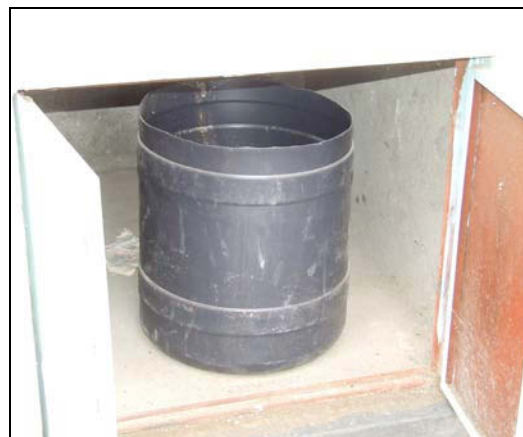
Figure 8 Faecal matter container inside the drying chamber
