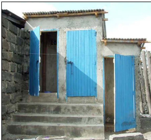
Figure 19 UDDT replication on a residential plot
