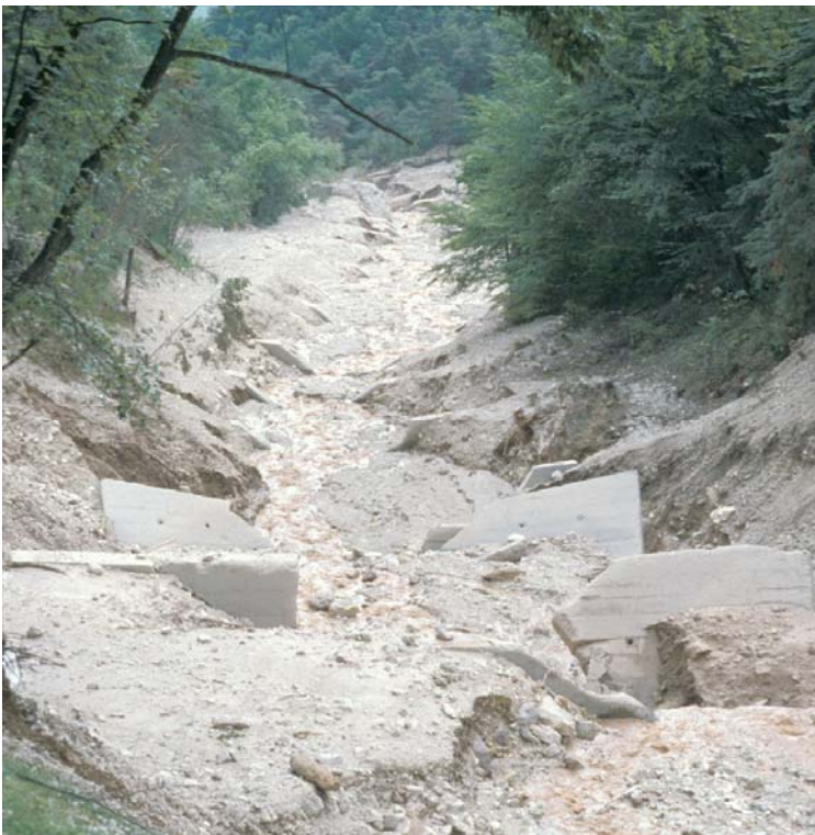
Figure 4-2. Toppling of a series of consolidation structures
