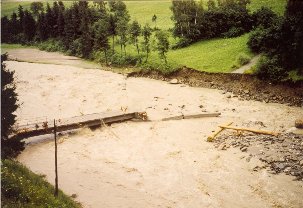
Figure 3-16: The figure shows the destroyed bridge across the Passer/Passiria river soon after the flood event in July 18th, 1987. The bridge was occluded with woody material and was destroyed after the outbreak of the river on the left side. The figure shows only the driftwood at the bridge that remained after the event.
