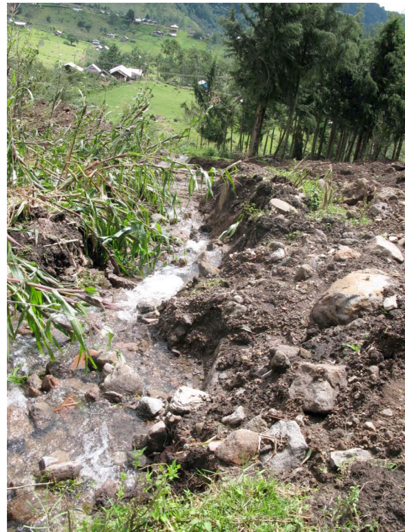
Figure 12 A small gorge caused by excess water runoff from the construction site.
