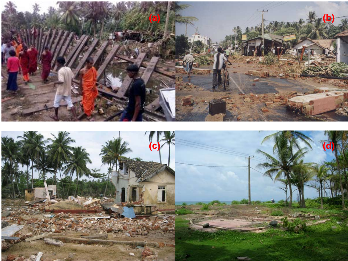
Figure 1.2: Damage caused by tsunami to the southern railway line (a), A-2 highway (b) and coastal houses (c) and (d); a few days (c) and 2 years (d) after tsunami
