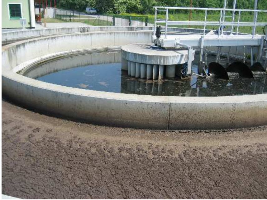
Fig. 5-39: One of the aeration and settlement tanks of the WWTP
