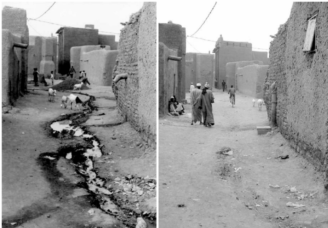
Figure 8: Street in Djenné: before implementation of the greywater infiltration trenches (left) and one year after implementation (right) (ALDERLIESTE and LANGEVELD, 2005)
