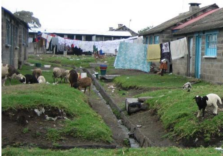
Figure 17: Stormwater (and greywater) drainage in a peri-urban settlement of Nakuru, Kenya (photo by LANGERGRABER, 2007)
