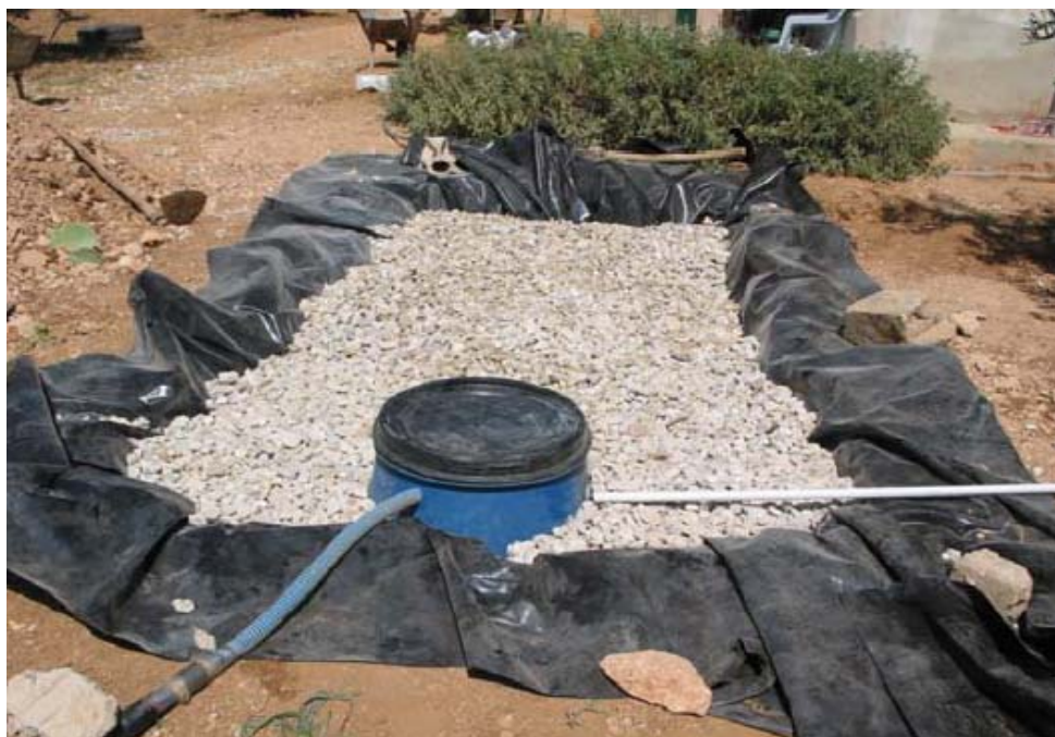
Figure 12: Confined trench greywater treatment system installed at a household in Jordan (AL-BEIRUTI, 2005)
