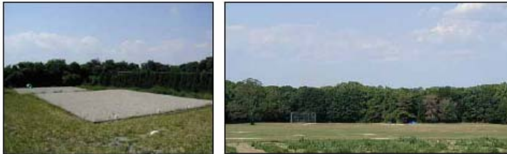
Figure 31: School recirculating media filter and the athletic practice field with the shallow narrow drainfield (Joubert et al., 2004)
