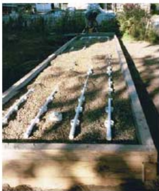
Figure 26: Bottomless sand filter following a recirculating media filter for multifamily and commercial use (Joubert et al. 2004).
