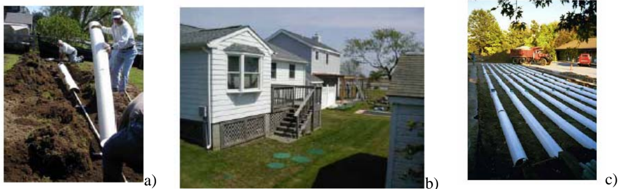
Figure 25: Shallow narrow drainfield - installation and application (Joubert et al. 2004)
