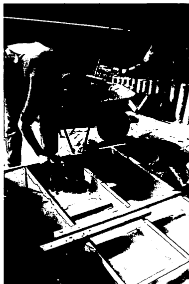
Picture 4.3.2-1 Casting of the concrete cover
