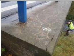
Fig. 20 ASR reaction on the concrete parapets
