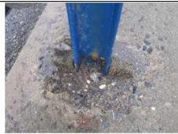
Fig. 21 Poor concrete of the parapets, safety barrier secured by timber
