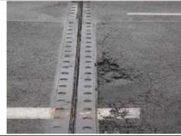
Fig. 17 The defects in the expansion joints and pavement nearby
