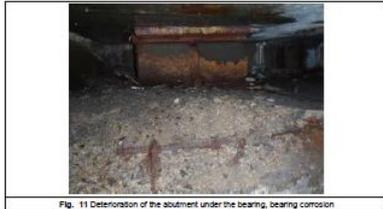
Fig. 11 Deterioration of the abutment under the bearing, bearing corrosion
