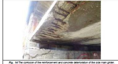
Fig. 14 The corrosion of the reinforcement and concrete deterioration of the side main girder.
