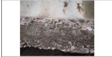
Fig. 15 The poor quality of the side main girder
