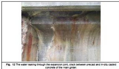
Fig. 12 The water leaking through the expansion joint, crack between precast and in-situ casted concrete of the main girder.
