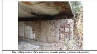
Fig. 10 Deterioration of the abutment – concrete spalling, reinforcement corrosion
