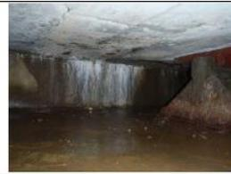
Fig. 18 The water leaking because of the expansion joint failure
