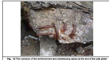
Fig. 13 The corrosion of the reinforcement and prestressing cables at the end of the side girder
