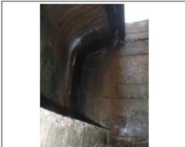
Fig. 19 The water leaking because of the waterproofing and expansion joint failure
