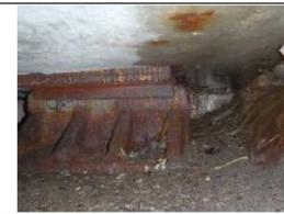
Fig. 22 The significant corrosion of the bearings
