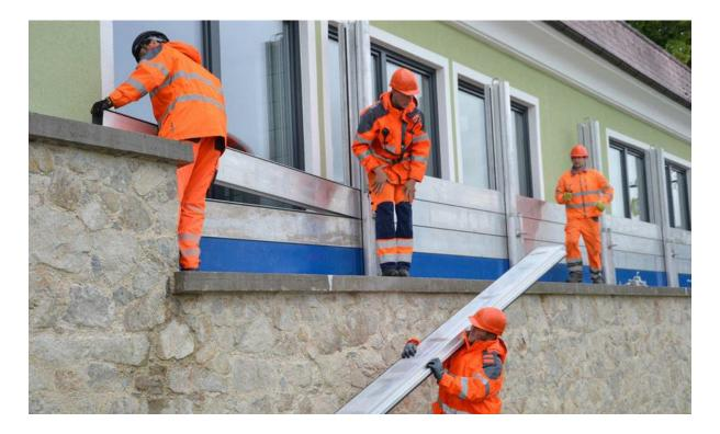
Figure 5: Construction of mobile water barriers for a house along the river Danube in Schärding, Upper Austria (from Habersack et al. 2015, p. 45).
