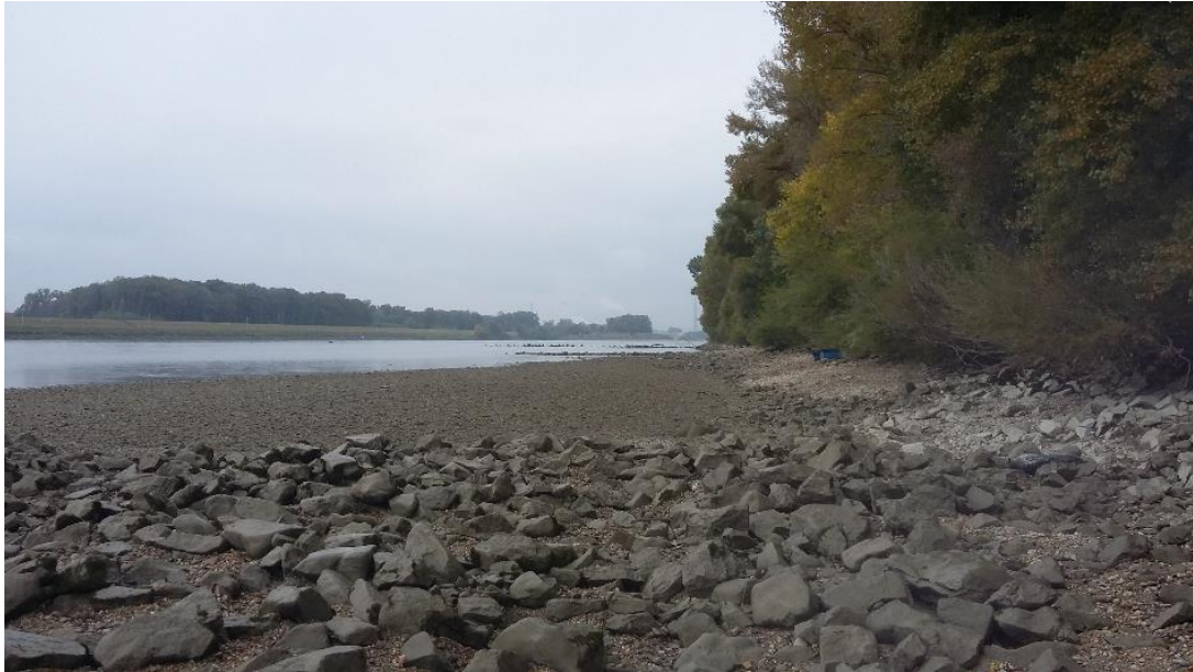
Figure 12: Rip-rap and groyne in the tailwater at Danube-km 1918.30, © Reisinger 2016
