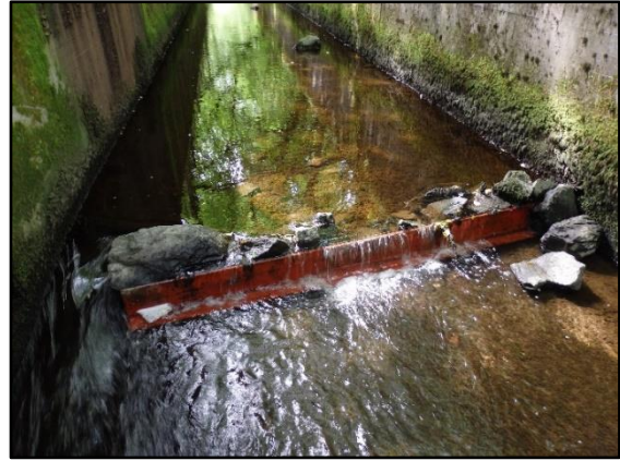
Figure 15: Metal bars and large stones to improve fish migration.
