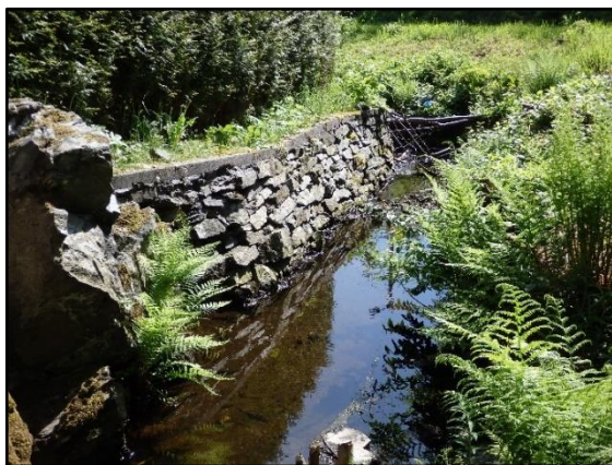
Figure 12: Bank stabilization in the form of a stone wall.
