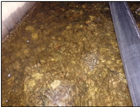
Figure 16: Substrate was placed in some culverts to improve the river bed's conditions.
