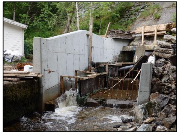
Figure 17: A fish ladder was installed to reestablish connectivity to the non-anadromous reach.
