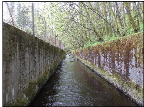
Figure 11: The concrete canal in study reach 1 essentially reduces habitat quality.
