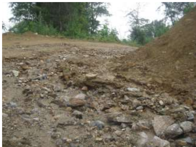
Photo 5: Erosion cannel formed due to surface runoff in the absence of side drains
