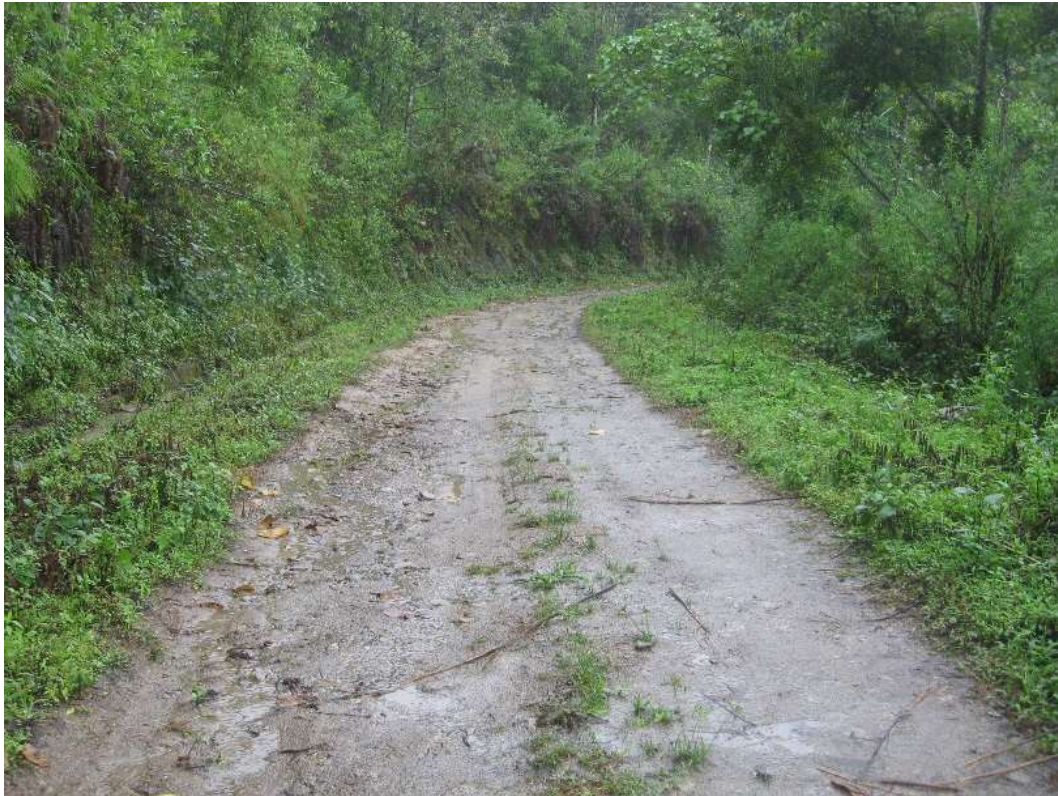
Photo 14: Naturally vegetated cut and fill slope
