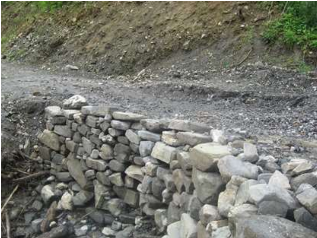
Photo 11: Locally made retaining walls
