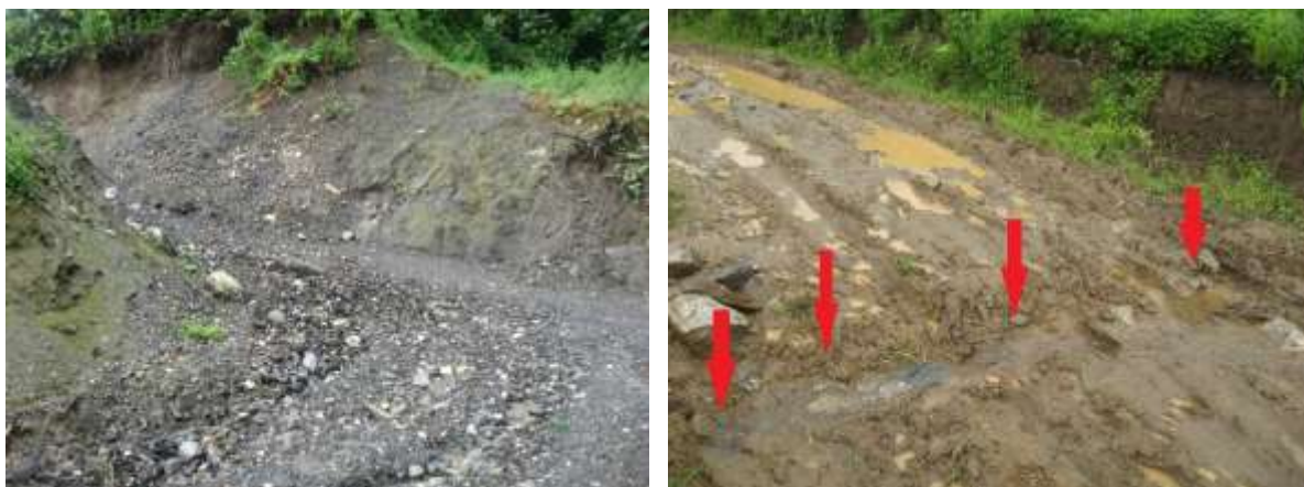
Photo 4: (Left) Road surface severely eroded due to runoff water on Gajeb farm road.(Right) Irrigation channels coming in conflict with the road alignment damaging the road surface
