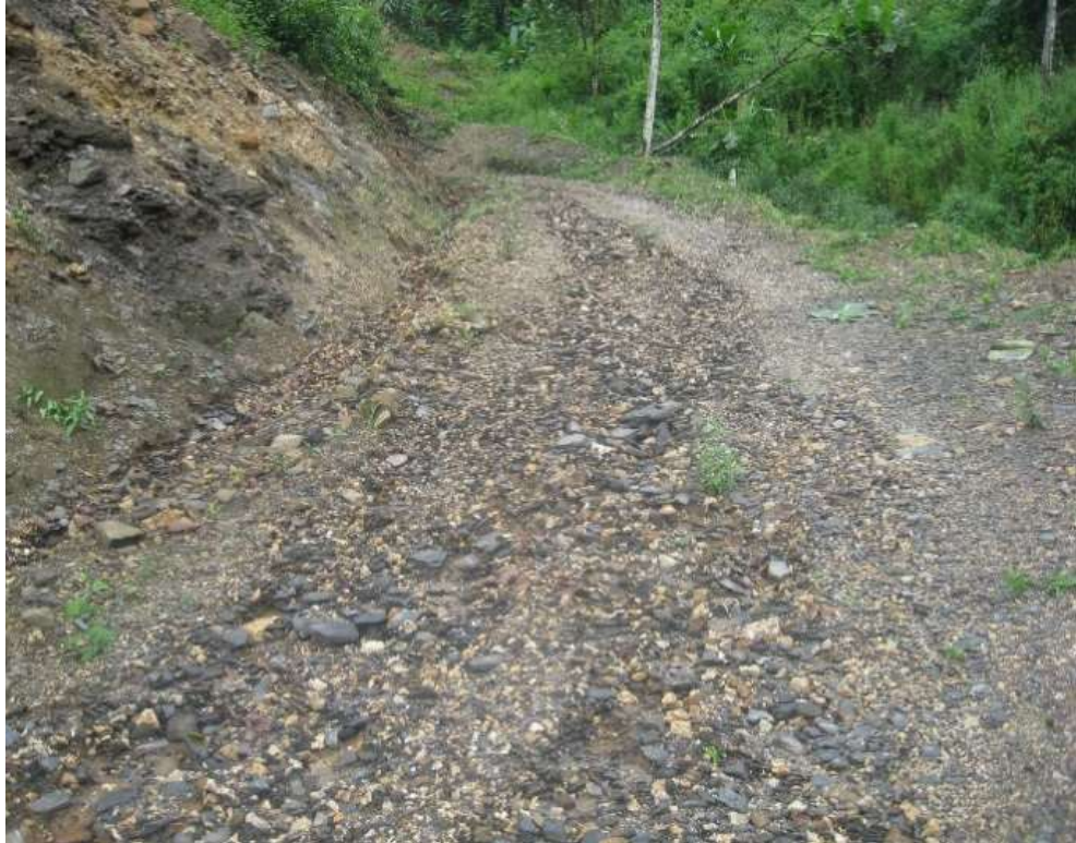
Photo 2: Road surface highly eroded due to steep road gradient (more than 7 degree or 12%)
