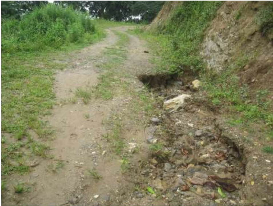
Photo 7: Deep erosion cannels formed on the road surface
