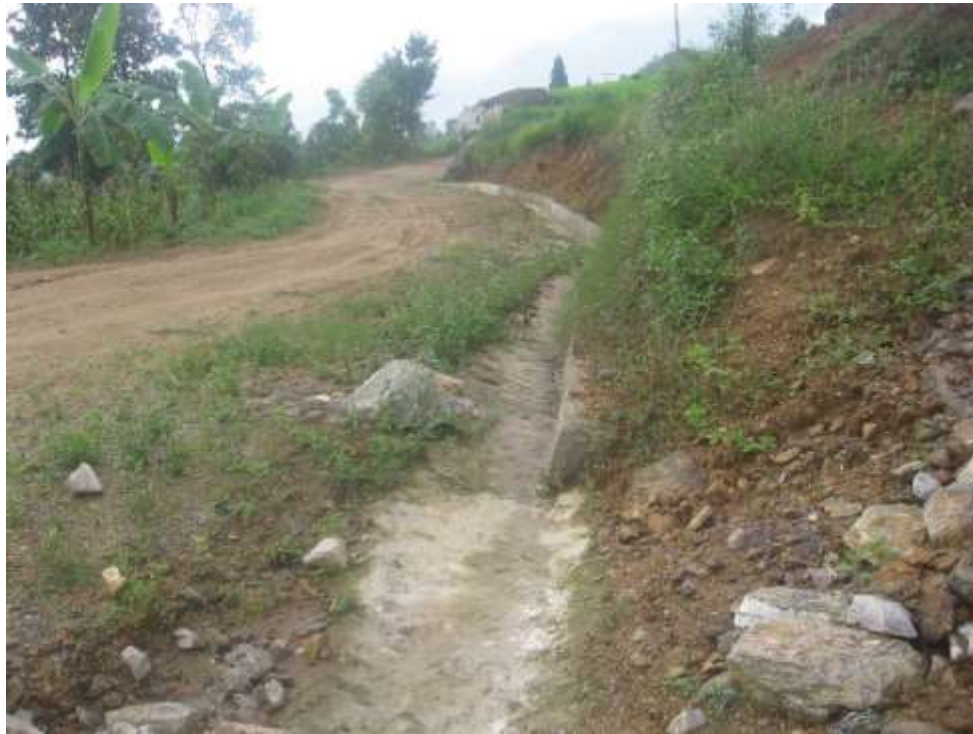
Photo 6: Side Drains for Goshi farm road in the watershed
