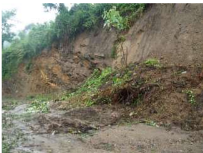
Photo 13: Erosion and road blocks due to cut slope failure
