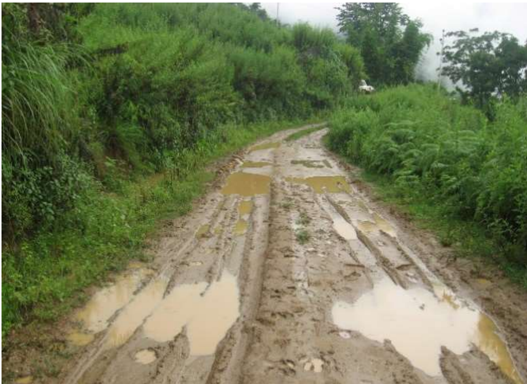
Photo 3: Water stagnation due to poor drainage and very low road gradient (less than 2 degree or 3%). Development of ruts on the road surface due to vehicle movements
