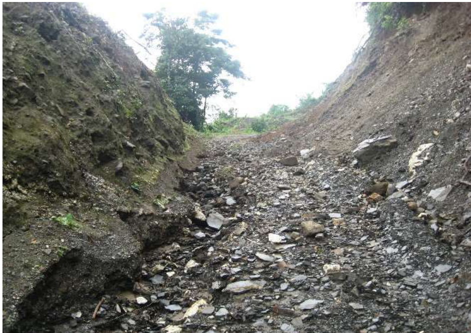
Photo 8: Road surface severely eroded due to excessive runoff
