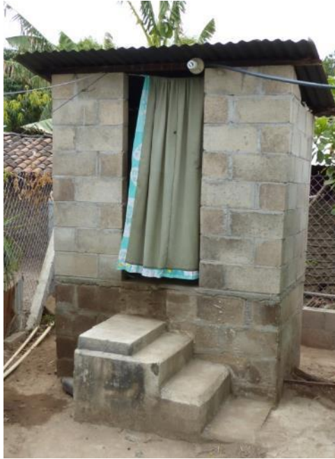
Figure 7: Dry latrine with two chambers
