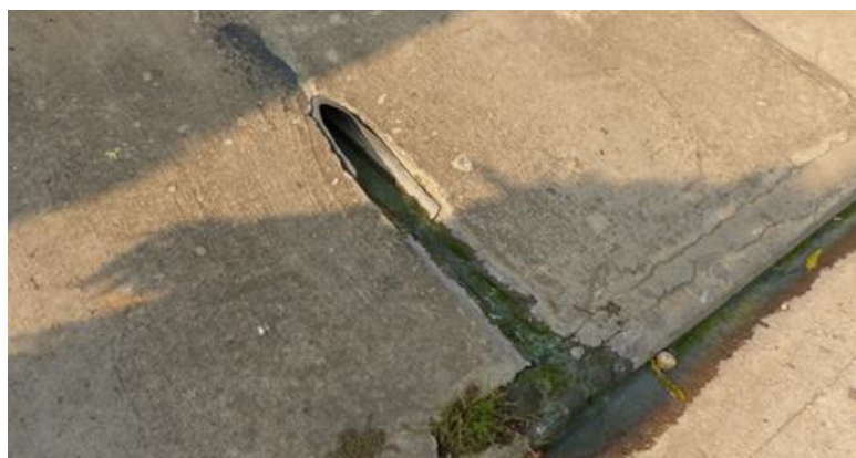
Figure 35: Typical discharge of grey water from households onto the street
