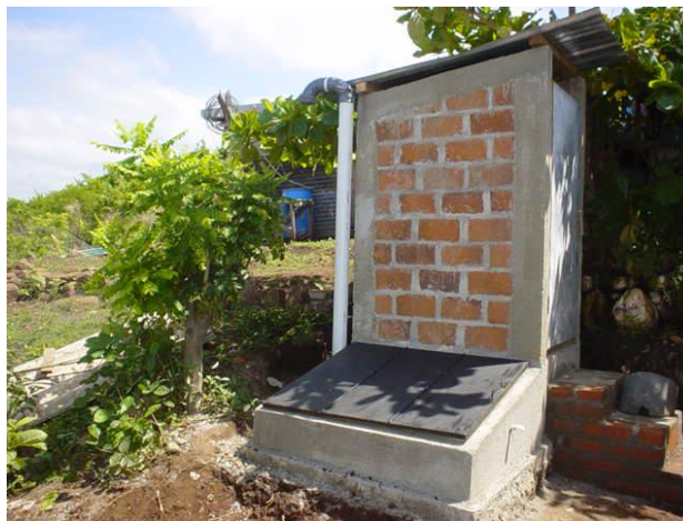
Figure 6: Dry latrine with solar drying (MINSAL, 2004a)
