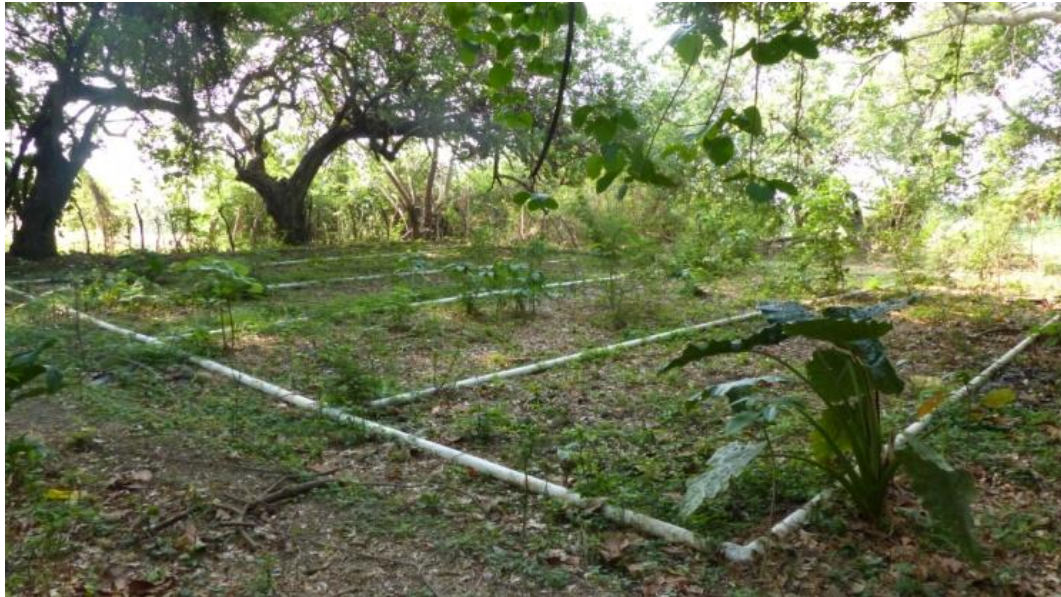
Figure 13: Uncontrolled vegetation on the first basin of the constructed wetland
