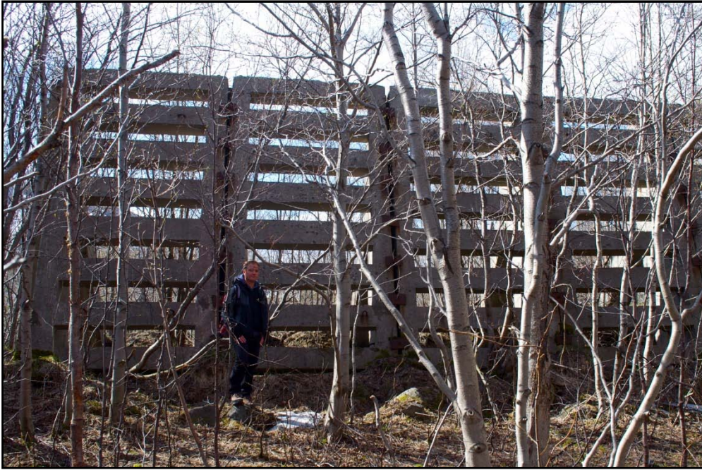
Figure 8: Concrete snow fences for the avalanche paths 13 and 14 (Pukhtel 2012)
