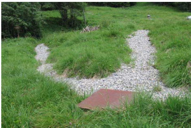
Figure 4-19. Enclosing structures: Drainage system to stabilise the sliding layers of the slope.
