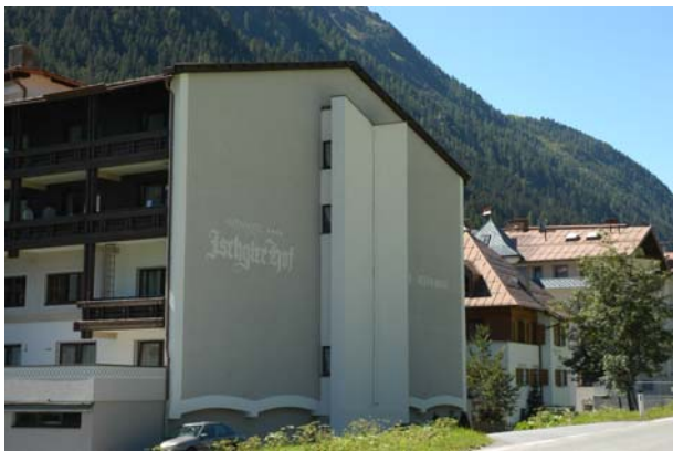
Figure 4-29. New building: Protection of windows by porched walls.
