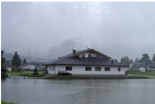
Figure 4-7. New building: Object built on altered (elevated) terrain (courtesy of: die.wildbach, 2005).
