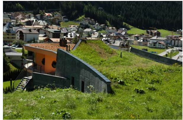
Figure 4-28. New building: Roof terrace to integrate the building into the surface of the slope.
