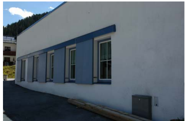
Figure 4-30. New building and upgrade: Window shutters to prevent intrusion of snow.
