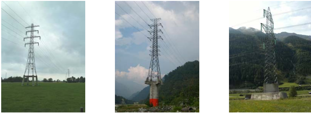
Figure 6-2. Strengthening of objects against flood at Netherlands (left), debris flow at Taiwan (middle) and dense avalanches at Austria (right). Source: middle by S. Fuchs
