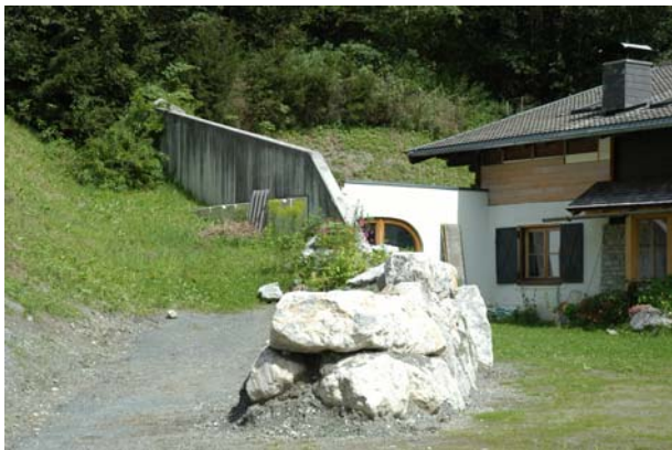
Figure 4-13. New building and upgrade: Deflection wall and dam.
