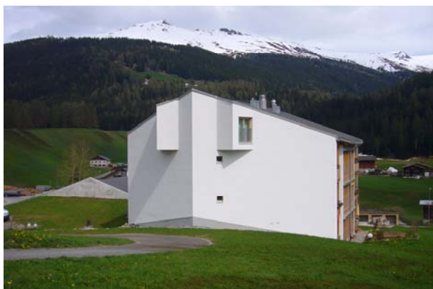
Figure 5-10. Splitting wedge directly connected to the exposed object (Davos Frauenkirch, Switzerland).
