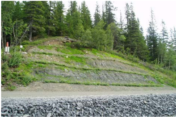
Figure 4-17. New building and upgrade: Soil bio-engineering measures to stabilise unsteady slopes (courtesy of: Rankka, 2005).
