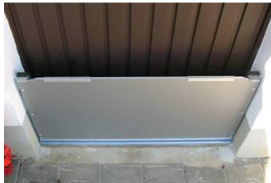
Figure 3-4. Sealing of openings by half-sided plates by magnet technique (WHS-Hochwasserschutzsysteme, 2007)
