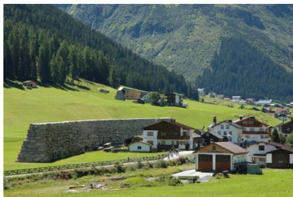
Figure 5-11. A deflection wall used to protect an entire building ensemble from the impact of medium-magnitude events (Galtür Tschafein, Austria)
