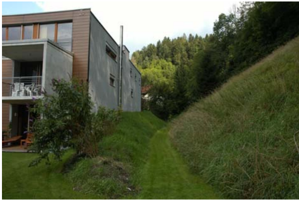
Figure 4-22. New building and upgrade: Earth-filled dam for energy dissipation of falling rocks.
