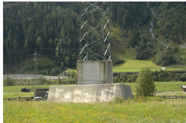
Figure 4-14. New building (and upgrade): Deflection wall and splitting wedge.
