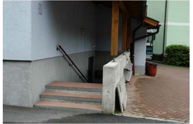
Figure 4-10. New building and upgrade: Enhancement (raising) of basement stairs above flood level.
