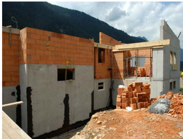
Figure 4-2. Brick walls reinforced by ferro-concrete components to strengthen the building's resistance.
