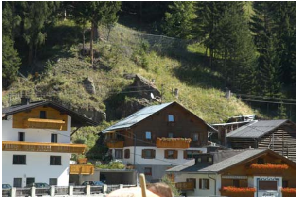
Figure 4-24. Enclosing structures: Net barrier to protect buildings against rock fall.
