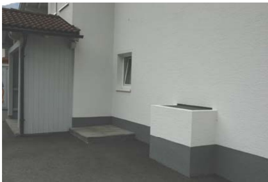
Figure 3-3. Enhancement (raising) of light wells above flood level
