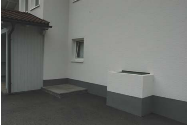
Figure 4-9. New building and upgrade: Enhancement (raising) of light wells above flood level.
