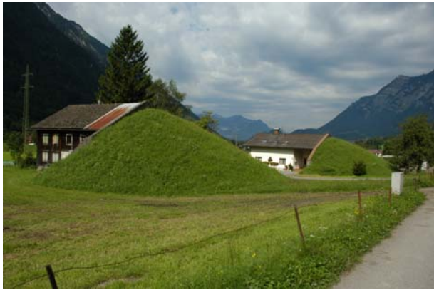
Figure 4-27. New building and upgrade: Earth-filled dams as deflection and splitting facilities.
