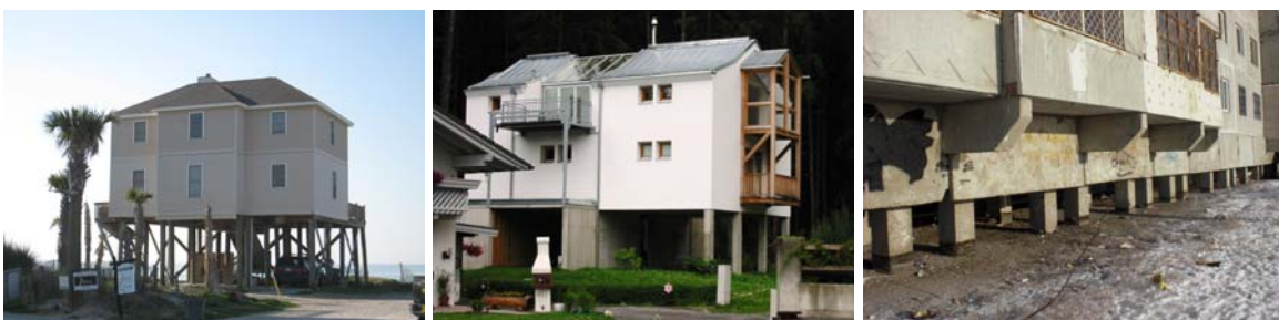
Figure 6-1. Elevated buildings for protection against water related hazards; spring tides at USA (left), torrent processes at Austria (middle) and permafrost-induced ground movement at Russia (right). Source: left and middle by S. Fuchs; right from http://bopohex.wordpress.com
