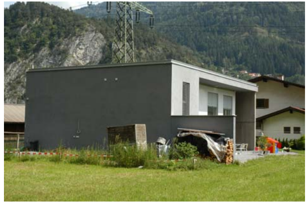
Figure 4-23. New building: Strengthened front wall without windows.
